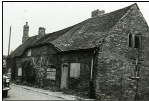
This is Mrs Bennett's cottage before demolition to build the new houses there on High Street
