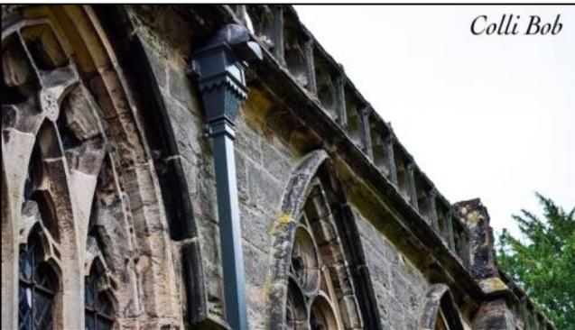
Finally some external works have been completed including lead roofing being sealed on the North aisle to prevent the current water ingress and the restoration of the hoppers and downpipes which are now looking fabulous, resplendent in their new grey paint.
